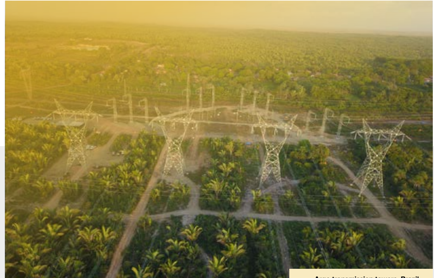
Argo transmission towers, Brazil
