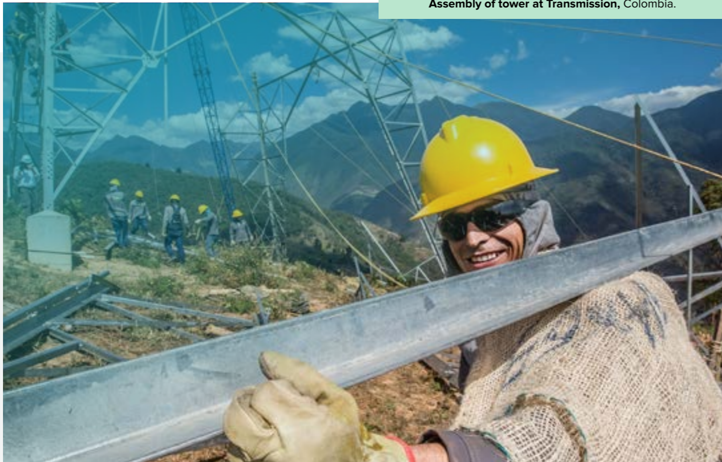
Assembly of tower at Transmission, Colombia.
